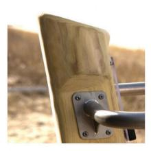
Construction made of Robinia - very durable acacia wood with a diameter of  $\sim 18$  cm without sharp edges, resistant to weather conditions,
